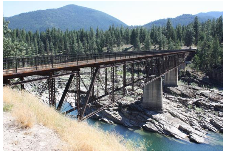
Thompson Falls High Bridge
